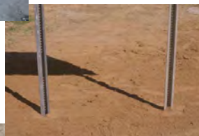
Fracturing Sign Support
