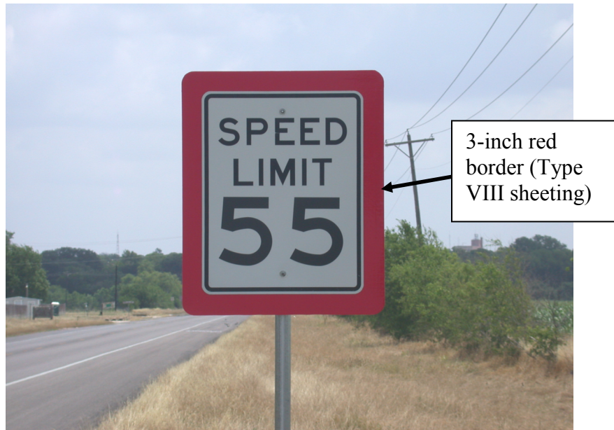
Figure 6. Speed Limit Sign (R2-1) with 3-inch Red Border.
