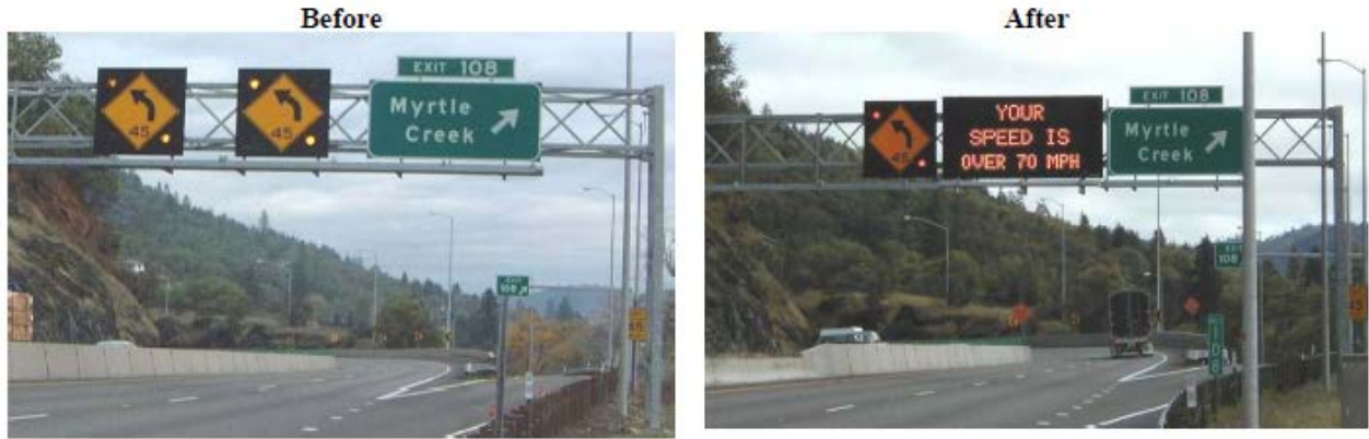
Figure 1. Photo. Northbound Interstate 5 DSFS systems in Oregon. (22)
