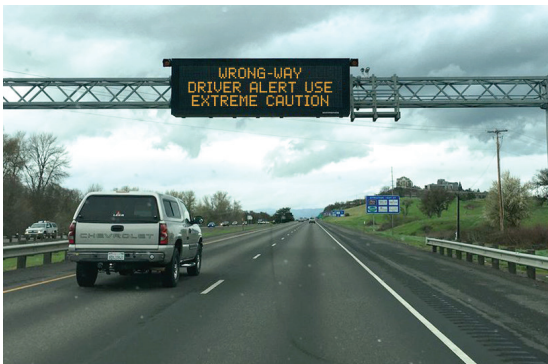
Warns right-way drivers on system-integrated overhead dynamic message boards
