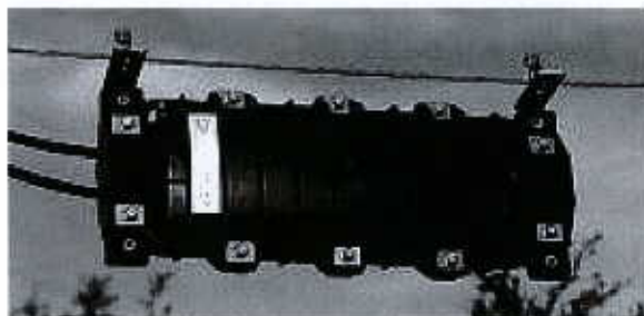
3M™ 2178-S case mounted on strand,
