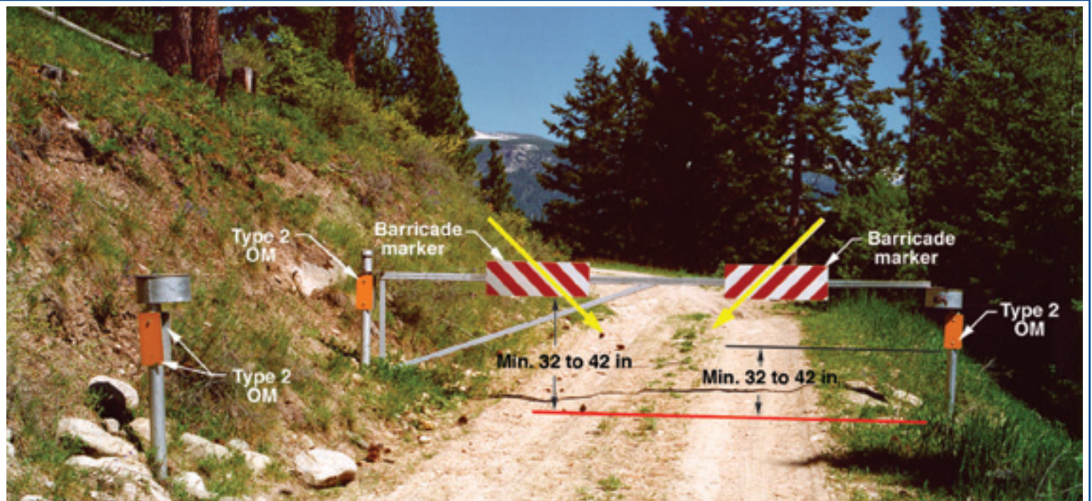
Gate Signing With Object Markers (OM) for One-Lane Roads
